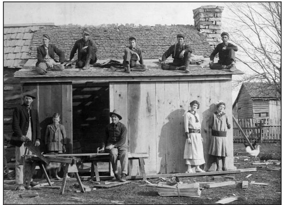
This appears to be a well dressed carpentry crew. This family is building an addition to the log cabin barely visible on the left side. Also barely visible in the lower left corner is a partial embossed imprint, "G. E. Ingram, Edgar Springs."
